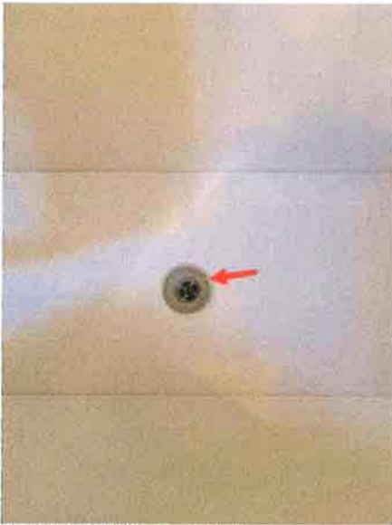
2nd Floor Bathroom Tub
